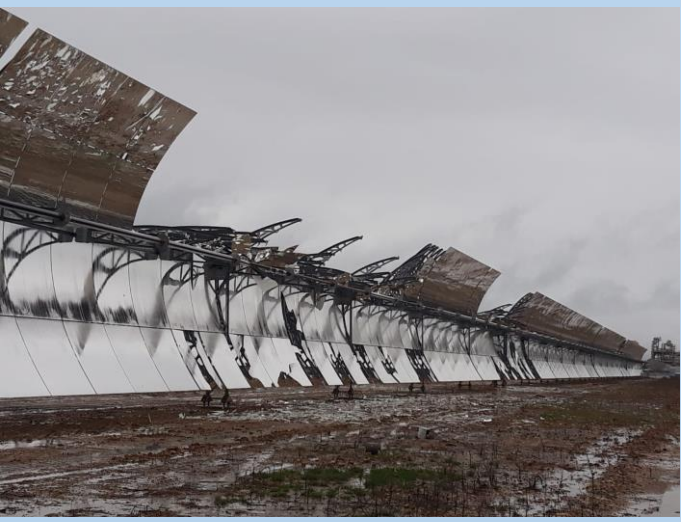
DI: SP (Solar Panels*) DoD: 0 (no structural failure) Rating: \leq IF1.5 ( \leq 180 km/h)
