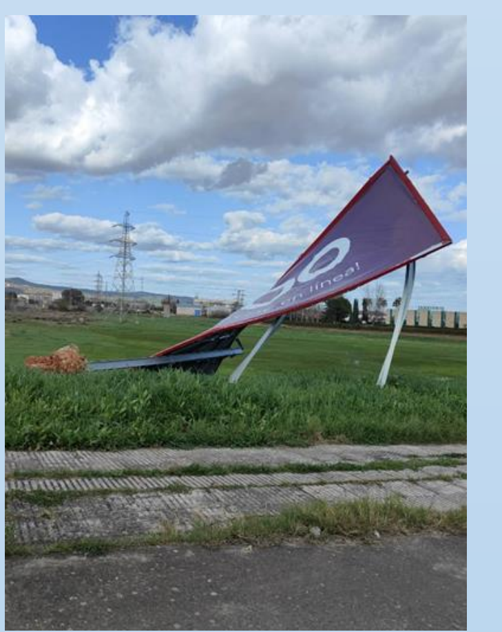
DI: SNM (metal frame billboard) DoD: 1 (inclination or buckling of pillars) Rating: IF1.5 (180 km/h)
