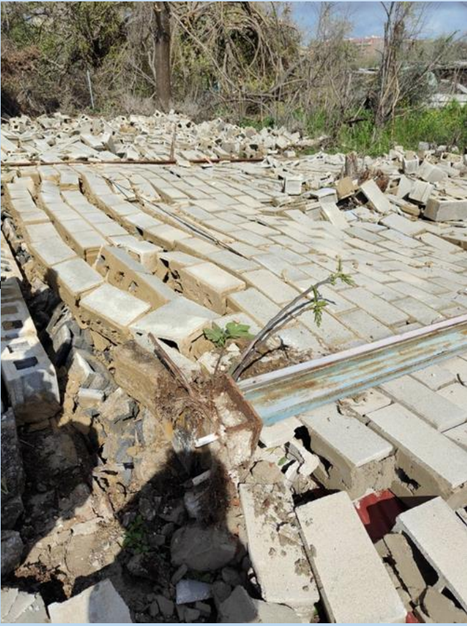
DI: FWAB (Free-standing Wall, concrete blocks reinforced) DoD: 2 (near complete destruction) Rating: \geq IF2 ( \geq 220 km/h)
