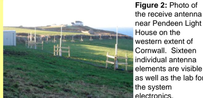
**Figure 2:** Photo of the receive antenna near Pendeen Light House on the western extent of Cornwall. Sixteen individual antenna elements are visible as well as the lab for the system electronics.
