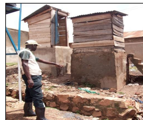
Elevated pit latrine unlined at the bottom
