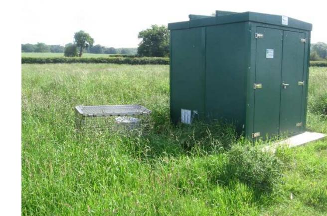
ISCO automatic samplers in bankside monitoring stations are remotely triggered to capture 1 litre stream water samples every 60-120 minutes during a storm, capturing the entire event in high-resolution.
