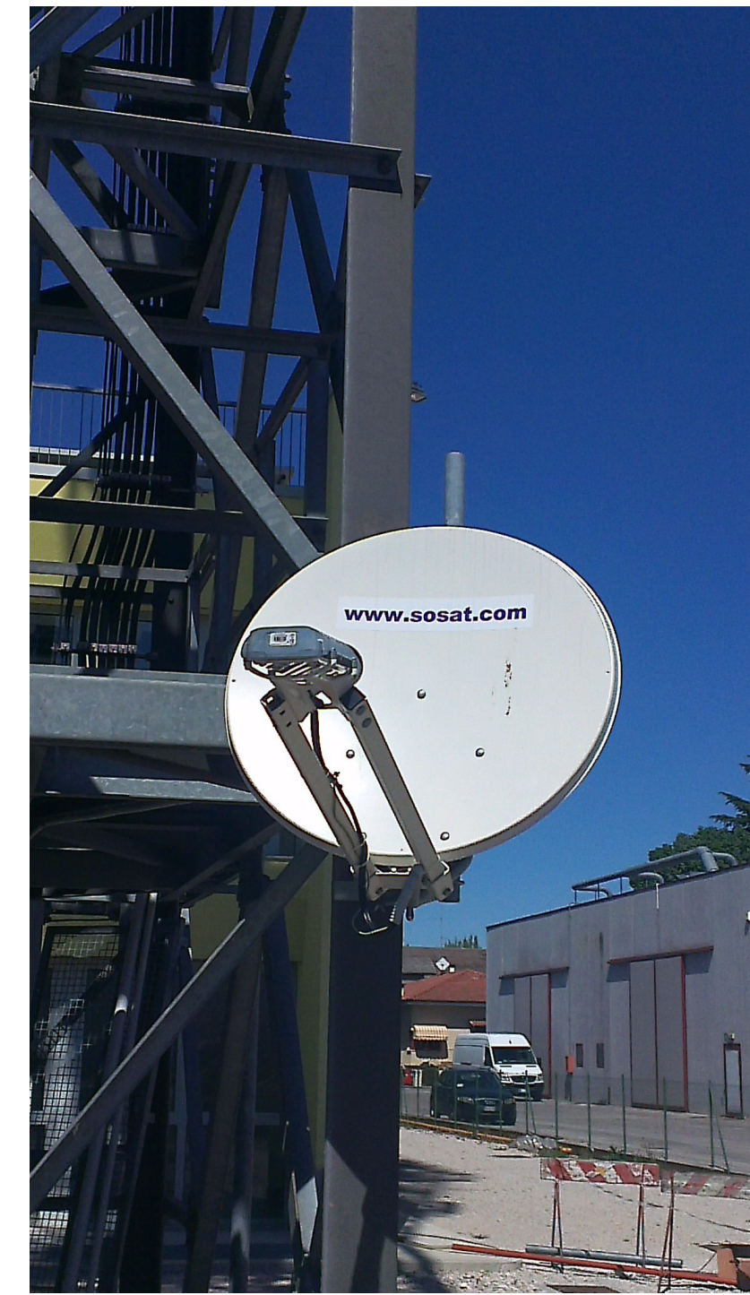
Fig. 4 - The Eutelsat KA-BA satellite terminal from the Austrian SOSAT ( http://www.sosat.at/ ) has been selected and is currently in testing phase. Its main characteristics are: • 18432kbit/s download, 6144kbit/s upload • 1 public IP address • 60GB data volume • Annual link availability >99,5% • RTTs Satellite round trip time < 600 ms • Lan/Ethernet Data Interface • Security: Time Division Multiple Access (TDMA)
