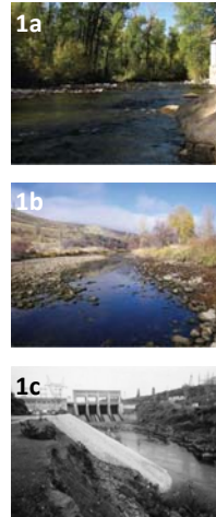
Figure 1: (a, b) river condition upstream and downstream the Echo Dam, Utah (USA); (c) sediment replenishment below Keswick Dam along the Sacramento river (USA) [photo by Kondolf G.M.]
