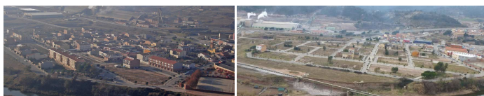
Figure 4. Image of Sallent site: 2010 view (left image) and 2015 view (right image) with most of the building demolished
