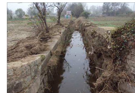
Figure 6. Detail of the small section of Riera de la Vall (a tributary of Sió) at Tarroja. It can convey 3 m 3 ·s -1 whereas the peak flow was 26 m 3 ·s -1 .
