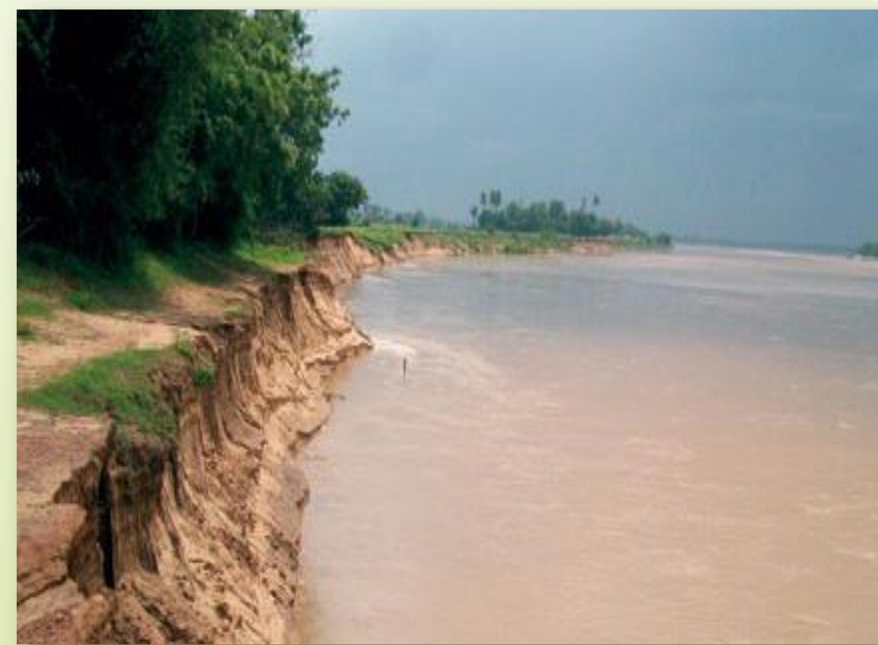
Figure 1: Bank erosion along the Mahanadi River. Source: The Telegraph, 2014
