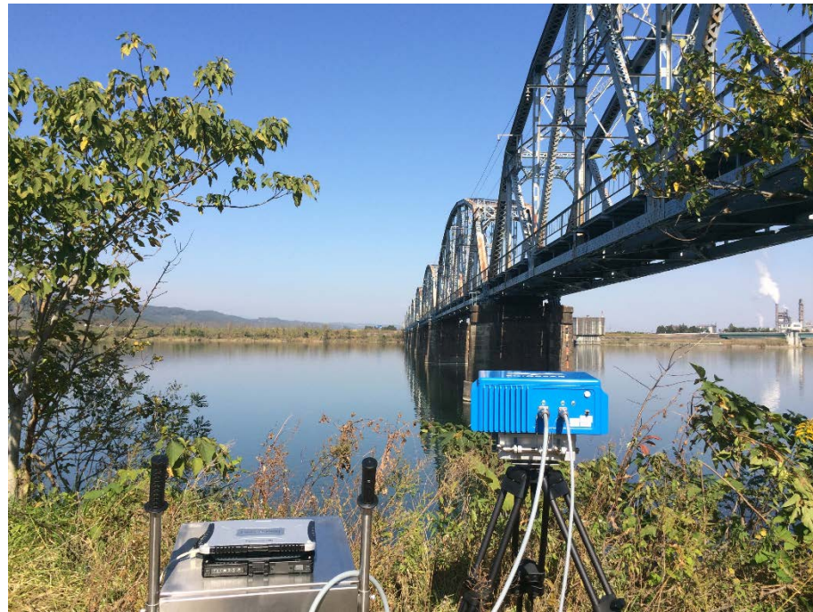
Bridge monitoring by polarimetric GB-SAR system (Sendai, Japan)
