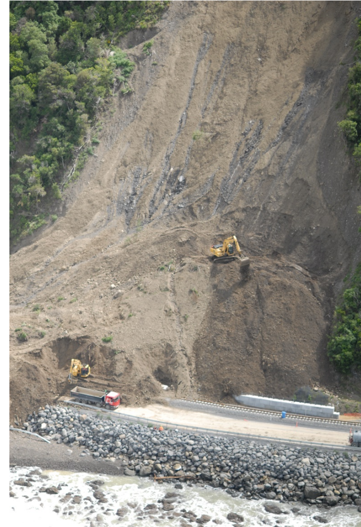
Debris flow deposit from reactivation of co-seismic landslide, SH1, Cyclone Gita, Feb 2018
