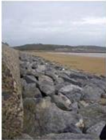
Rip Rap (Rock Armour)
