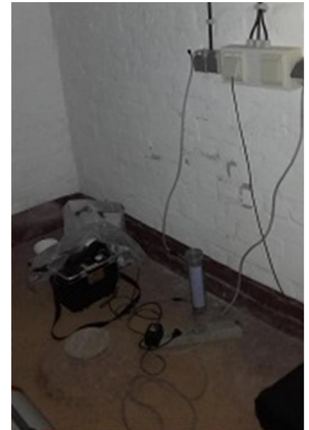
measurements radon concentration in air by using RAD7 detector in server room
