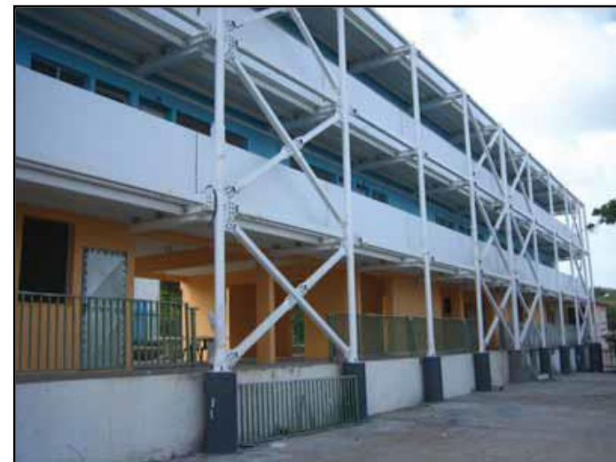
Structural reinforcement of a school in the Lesser Antilles (most exposed area to earthquakes in France) partly financed by FPNRM.
