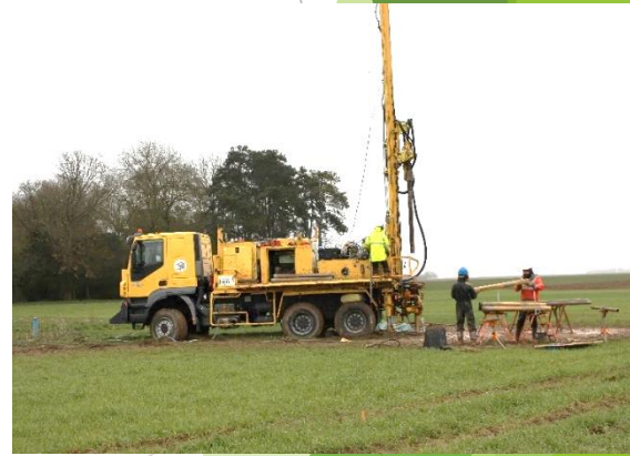
Boreholes drilling in O-ZNS site (25/02/2020)
