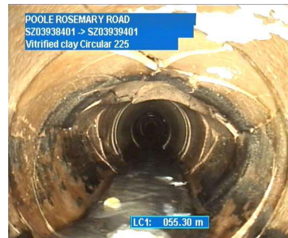
Collapsed Pipe
