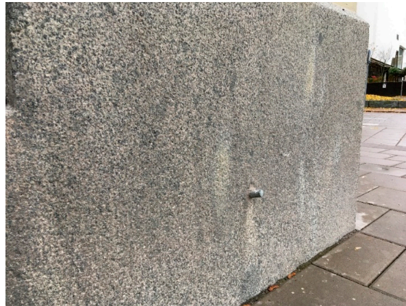
Figure 3. A metal peg, that has been measured with precise leveling, mounted in a building's foundation (photo: Jonas Fryksten).
