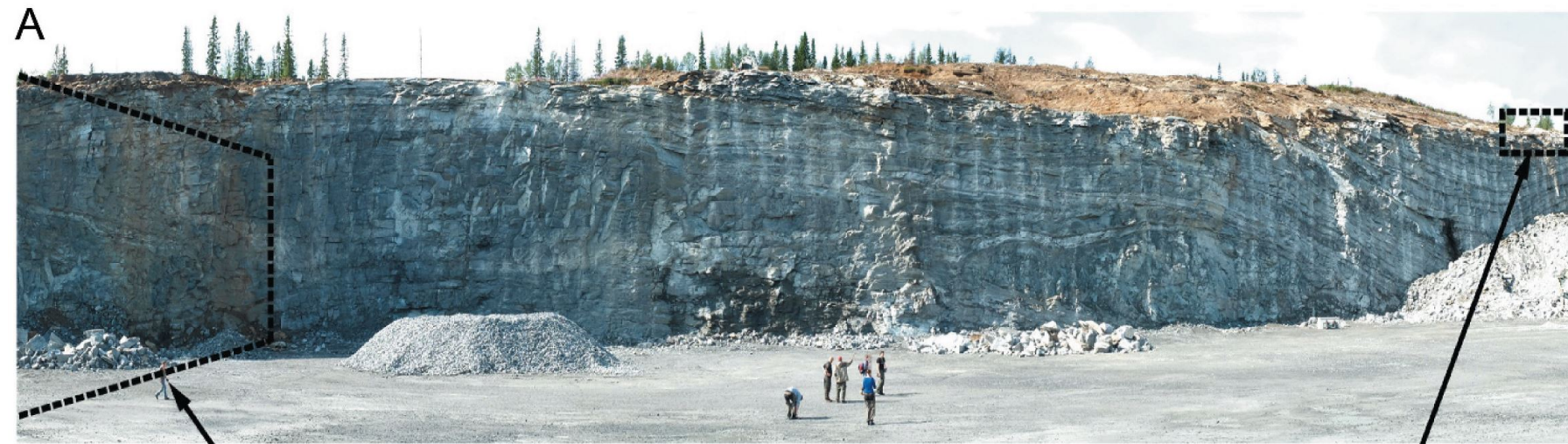
A. Looking south at the main face.
