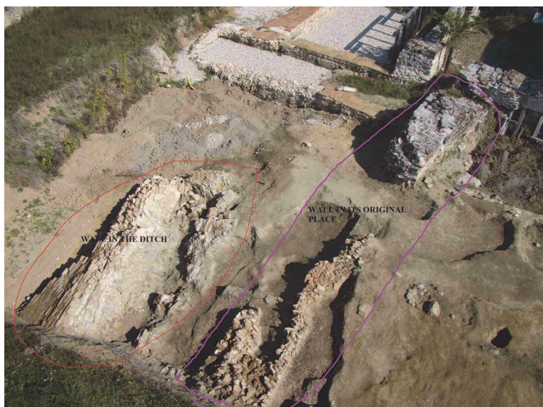
Figure 2. A collapsed segment of the city wall of Roman Siscia. There are still low parts of the wall in place on the right. Top of these walls displays clear sign of shearing to the left. Upper portion of the wall is in the city moat on the left: brick layers are bottom-up(!). North to the left
