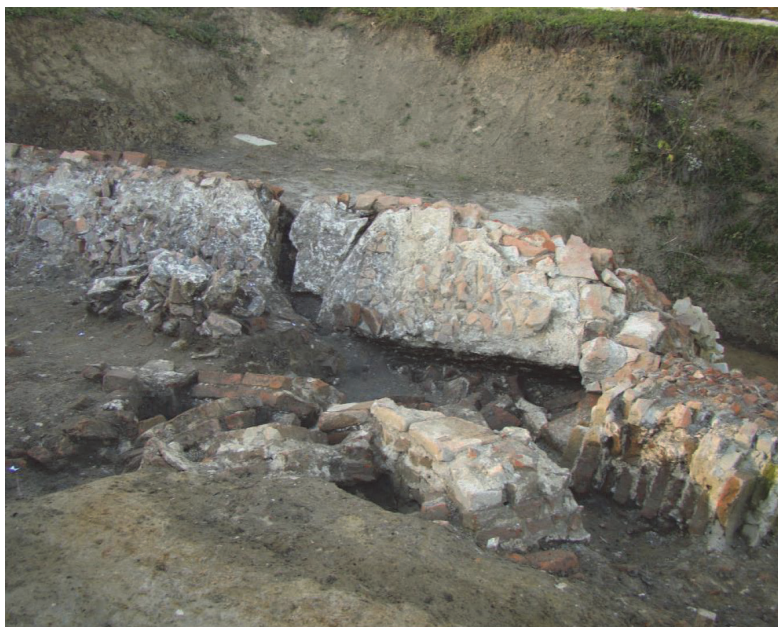
Figure 3. Overturned wall in the moat. The viewer is looking at a mortar layer between rows of bricks, a seen from below(!). Note that in-plane deformation caused a wide gap to appear, marking extension of the wall during shaking or during collapse [37]
