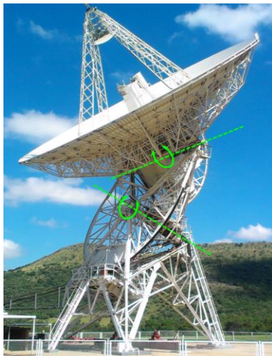
Fig.7 26m VLBI antenna axes
