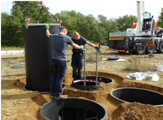
Installation of new HDPE columns
