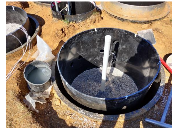
Filling of columns and installation of electrical resistivity sensors
