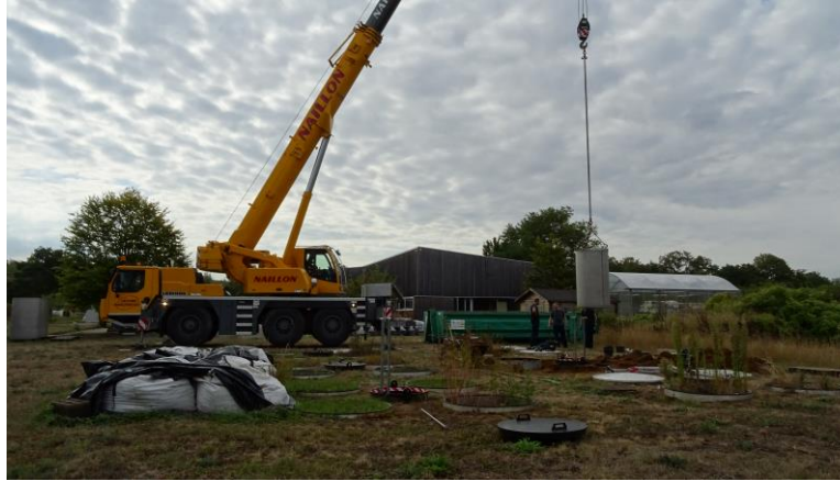
Removal and emptying of old columns
