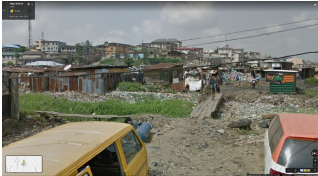
Drainage channel blocked by waste. Source: Google Street View.
