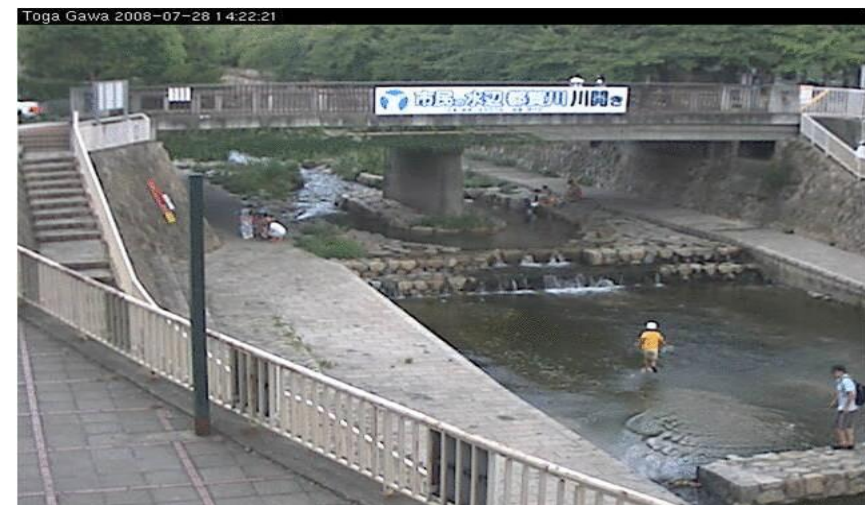
Flash Flood occurred during 30 min caused by Guerrilla heavy rainfall
