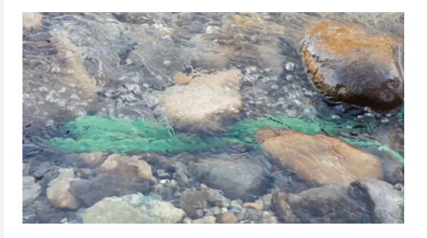
The tubing was attached to the riverbed and covered the entire width of the riverbed
