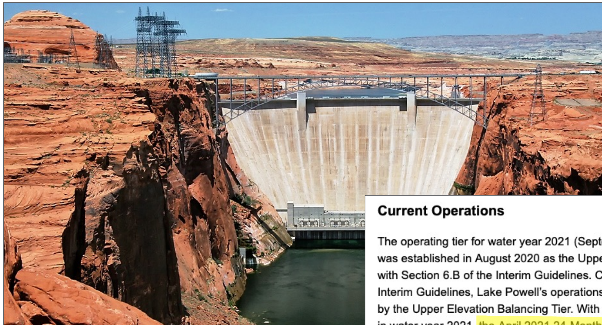
Glen Canyon Dam
