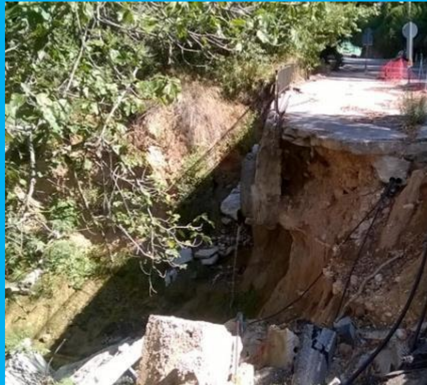
View from the slope failure (fall) of the examined road (Directorate of Technical Works/Region of Attica, 2020)
