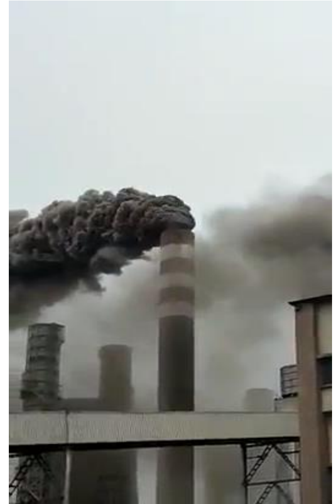
Afşin Elbistan Power Plant – May 2022
