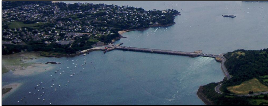
The sea wall (barrage – La Rance, France 1966 – 240 MW peak power)
