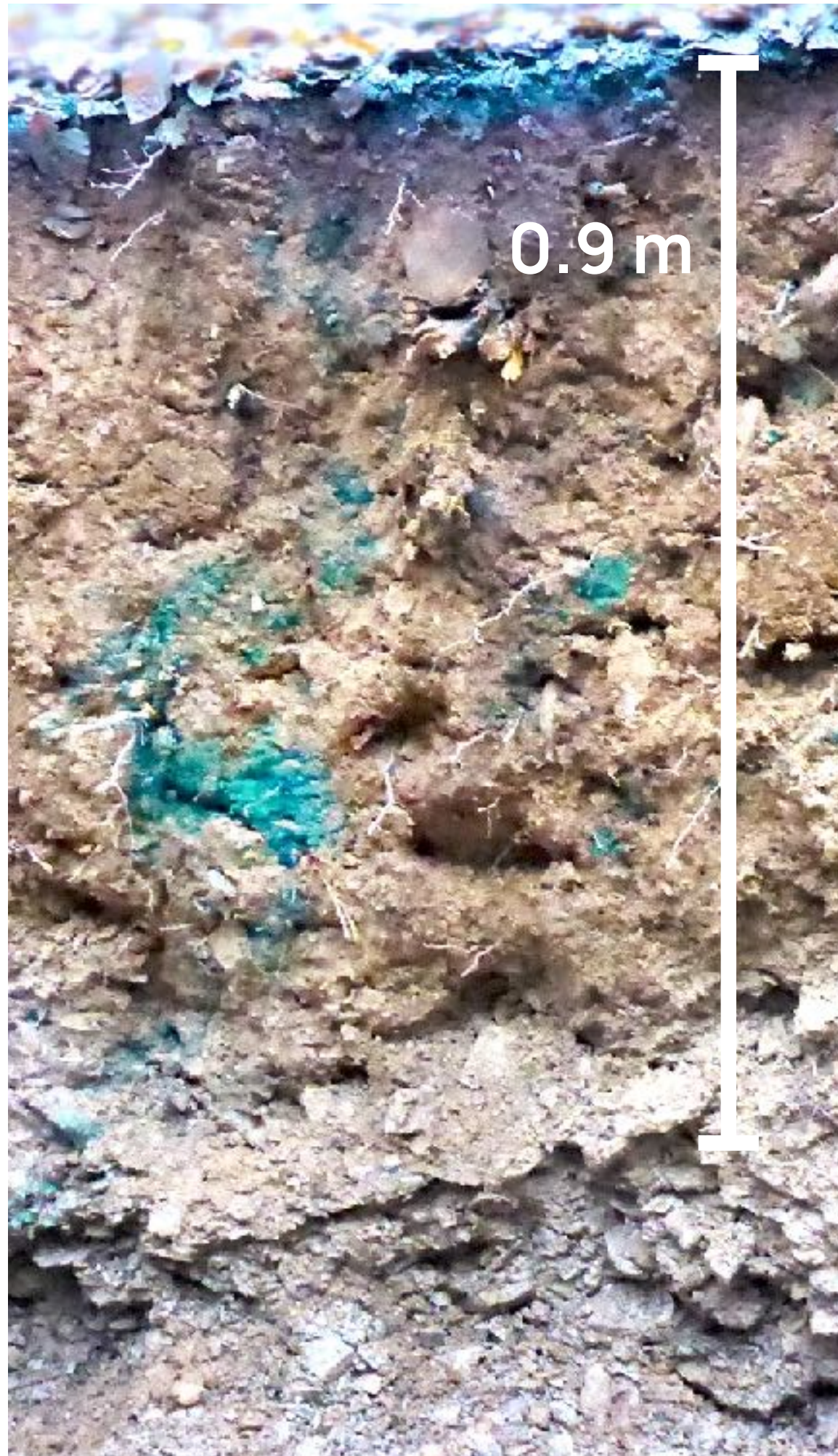
Silty soil slate slopes
