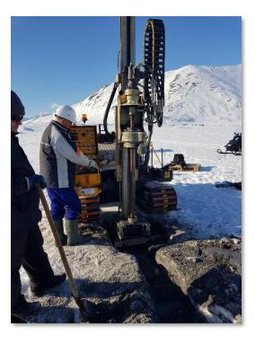
Three boreholes with continous thermal monitoring down to 5, 10 and 20 m.
