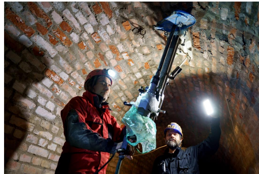
Validation by drilling.
