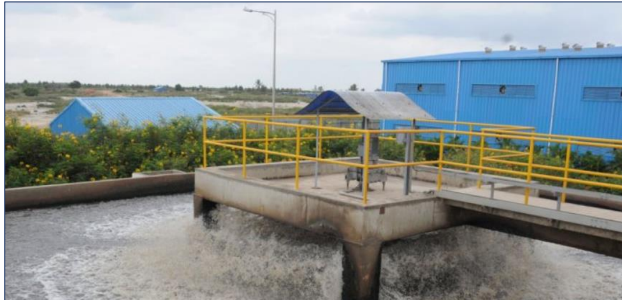
KC valley 55 MLD unit with blowers for air supply
