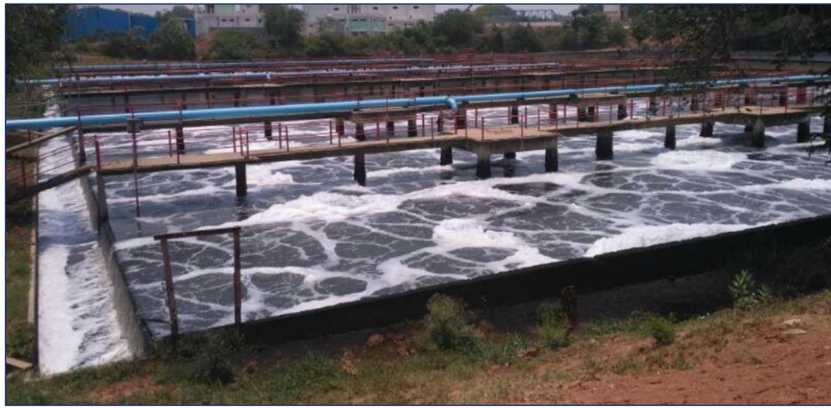
KC valley 55 MLD unit with blowers for air supply
