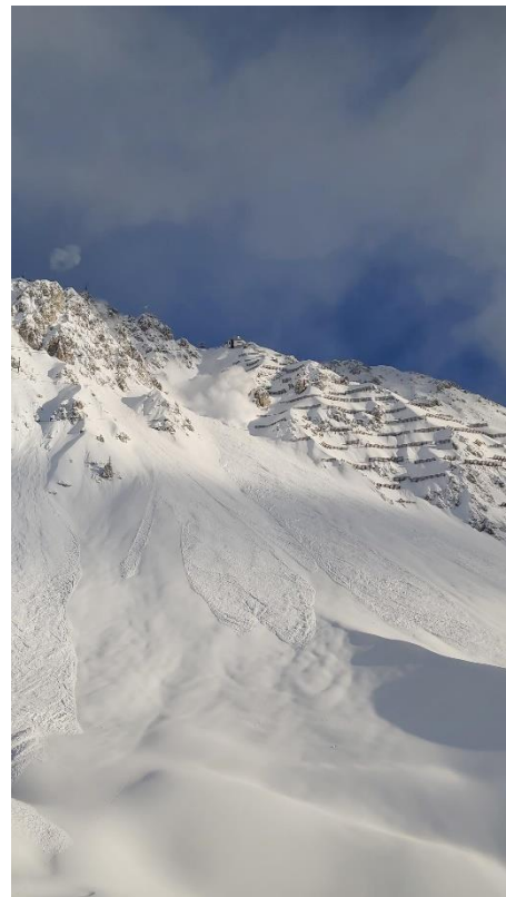
Fig.9: Seilbahnrinne View from bottom
