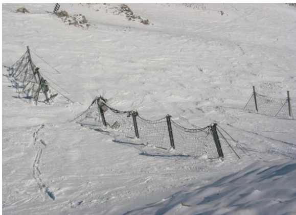
Fig.2: Snownets at Hafelekar, Innsbruck, Austria.
