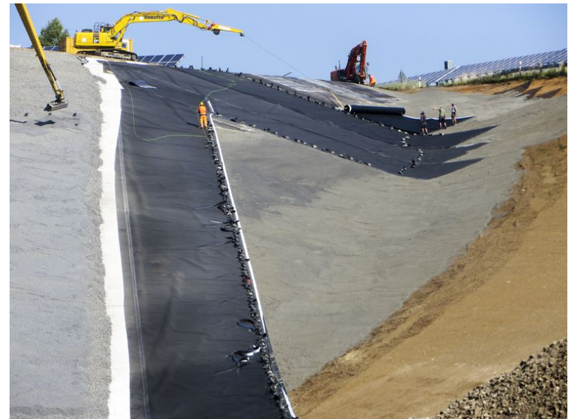
Installation of the HDPE liner by using a long arm excavator [ https://www.agru.at/ ]
