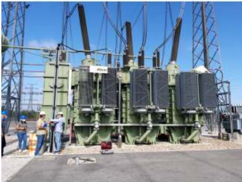
Installation of the sensor at Paraimo substation on the TRF6 transformer.
