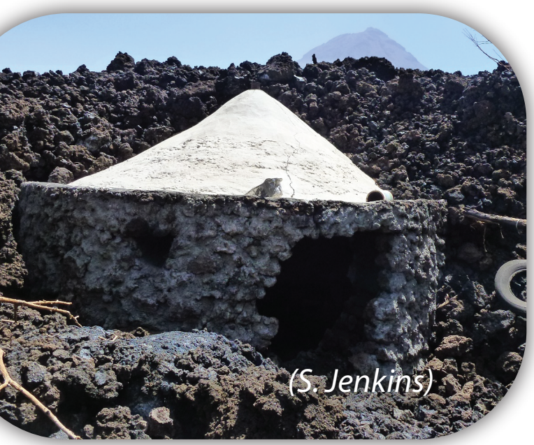
Above: Circular structure remains intact in contact with lava during the 2014-2015 Fogo lava flows, Cabo Verde.
