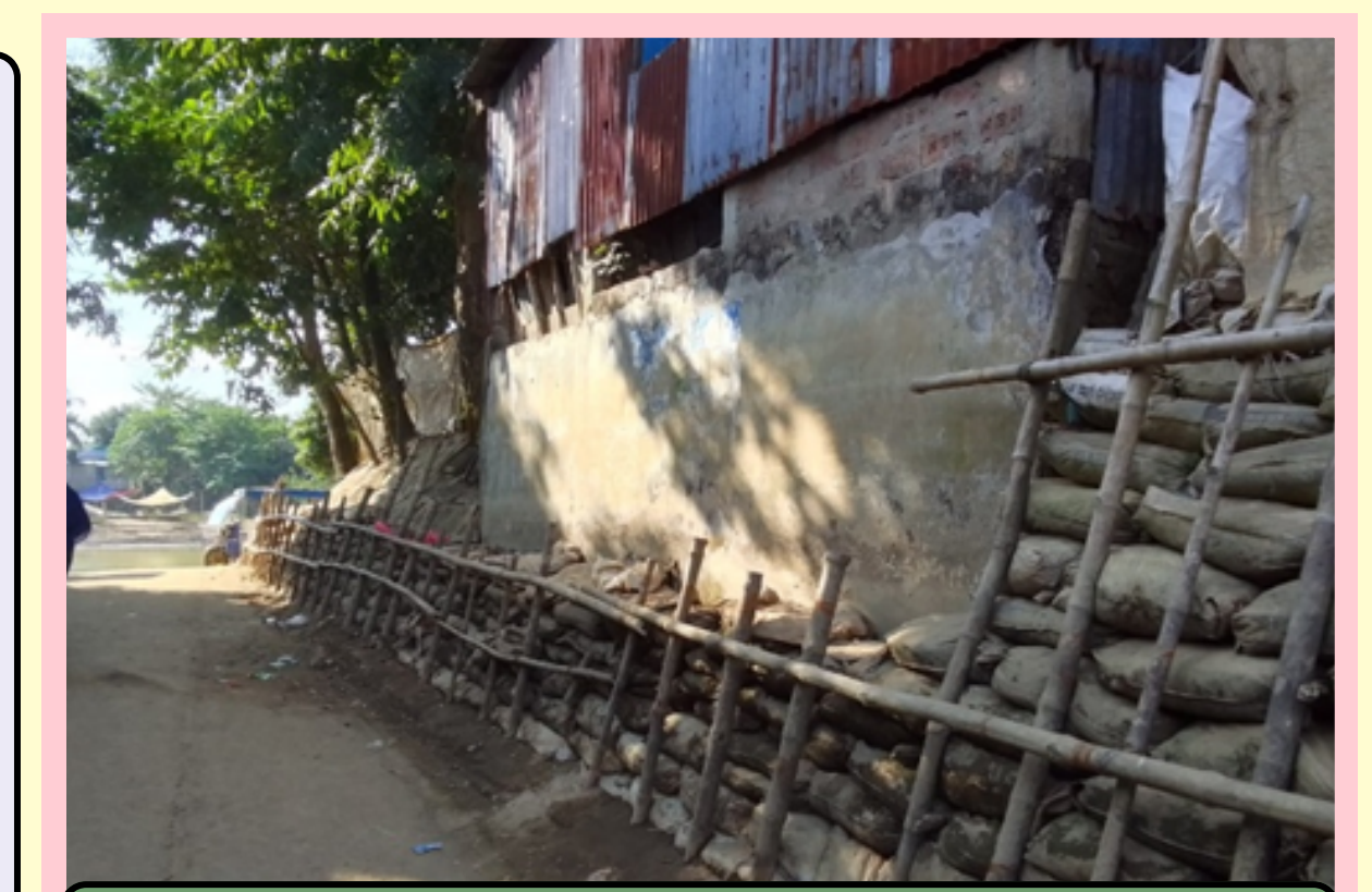
Fig 05: Increasing Plinth Level
