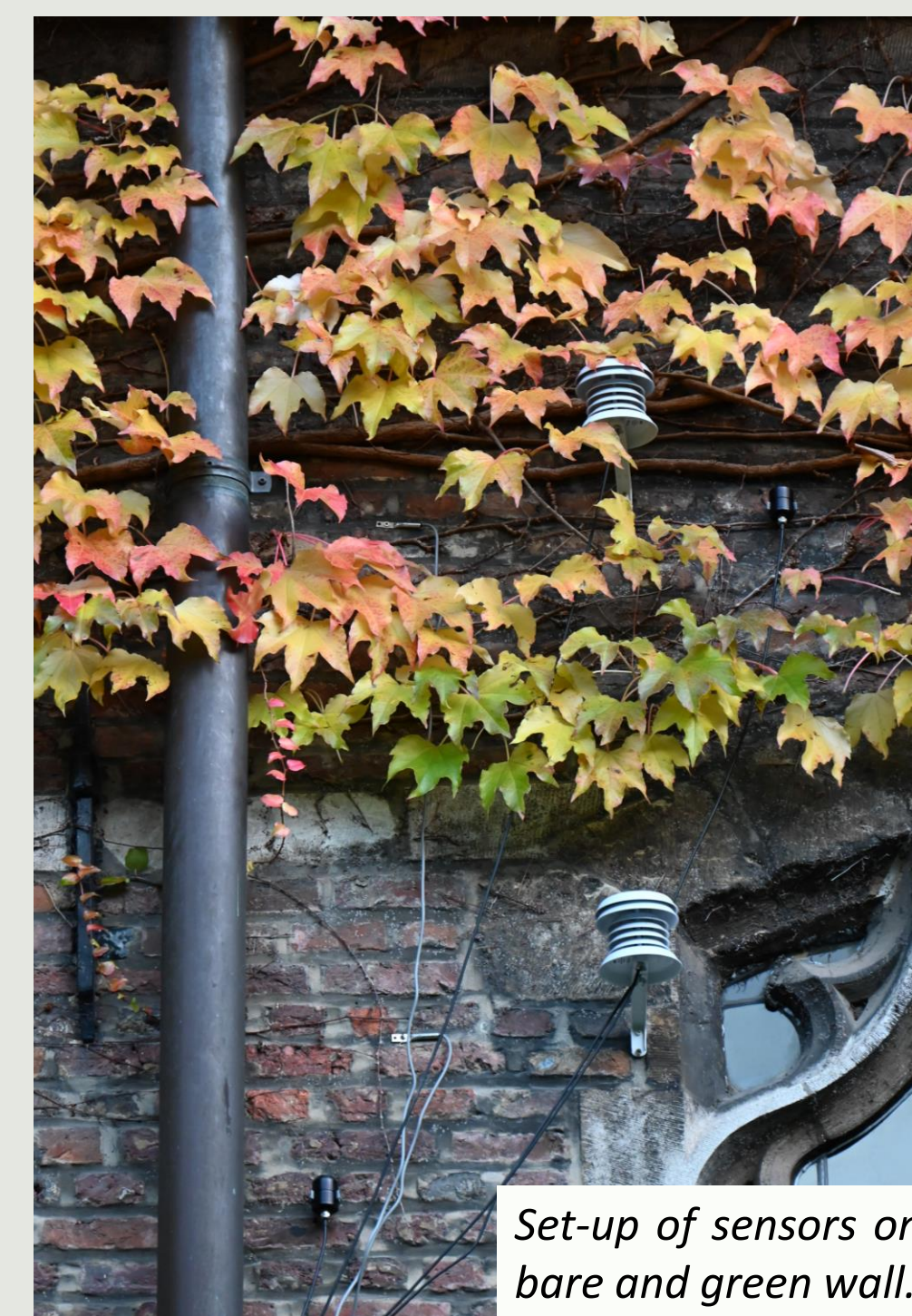
Figure of case study: Courtyard 'Hof Van Liere' in Antwerp, Belgium. The vegetation consists of a mature deciduous Virginia Creeper.
