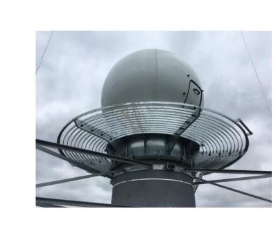
An X-band Doppler weather radar with dual polarization (GMWR-25-DP by GAMIC) for precipitation research has been in operation since autumn 2022. The weather radar is installed on the roof of the historical water tower (Institute of Meteorology, Freie Universität Berlin) on the Fichtenberg in Berlin-Steglitz. The weather radar has a range of 100 km.
