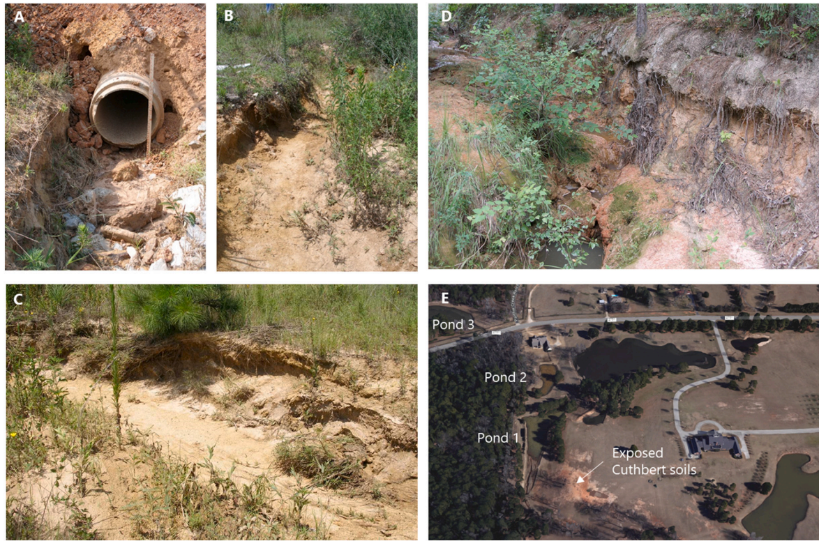
Fig. 4. Photographs of erosional features on both the defendant's and plaintiff's properties. (A) at the culvert along the western boundary of the defendant's property (see Fig. 1); (B) looking downstream from photograph A; (C) the gully northwest of the storage facility (see Fig. 1); (D) an incised channel on Cuthbert soils proximal to Pond 1; (E) aerial image looking east toward the ponds showing exposed Cuthbert soils on the plaintiff's property.
