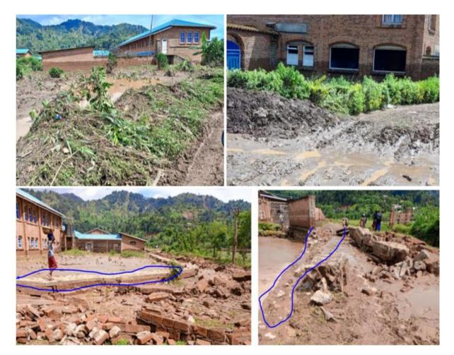
Nyundo Minor Seminary School in Rubavu District. Photos taken on 5th May 2023; the blue line to the left indicates the location of a masonry brick wall and to right the stone masonry foundation destroyed by water during the flooding (Hahirwabasenga et al., 2024).
