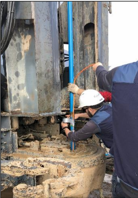
Electrodes array installed in PITOP5
