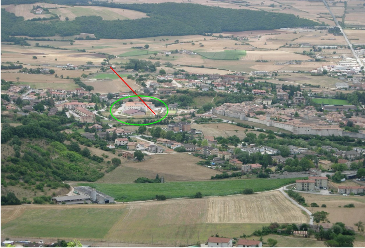
Trace of the FAC interfering with the school building.
