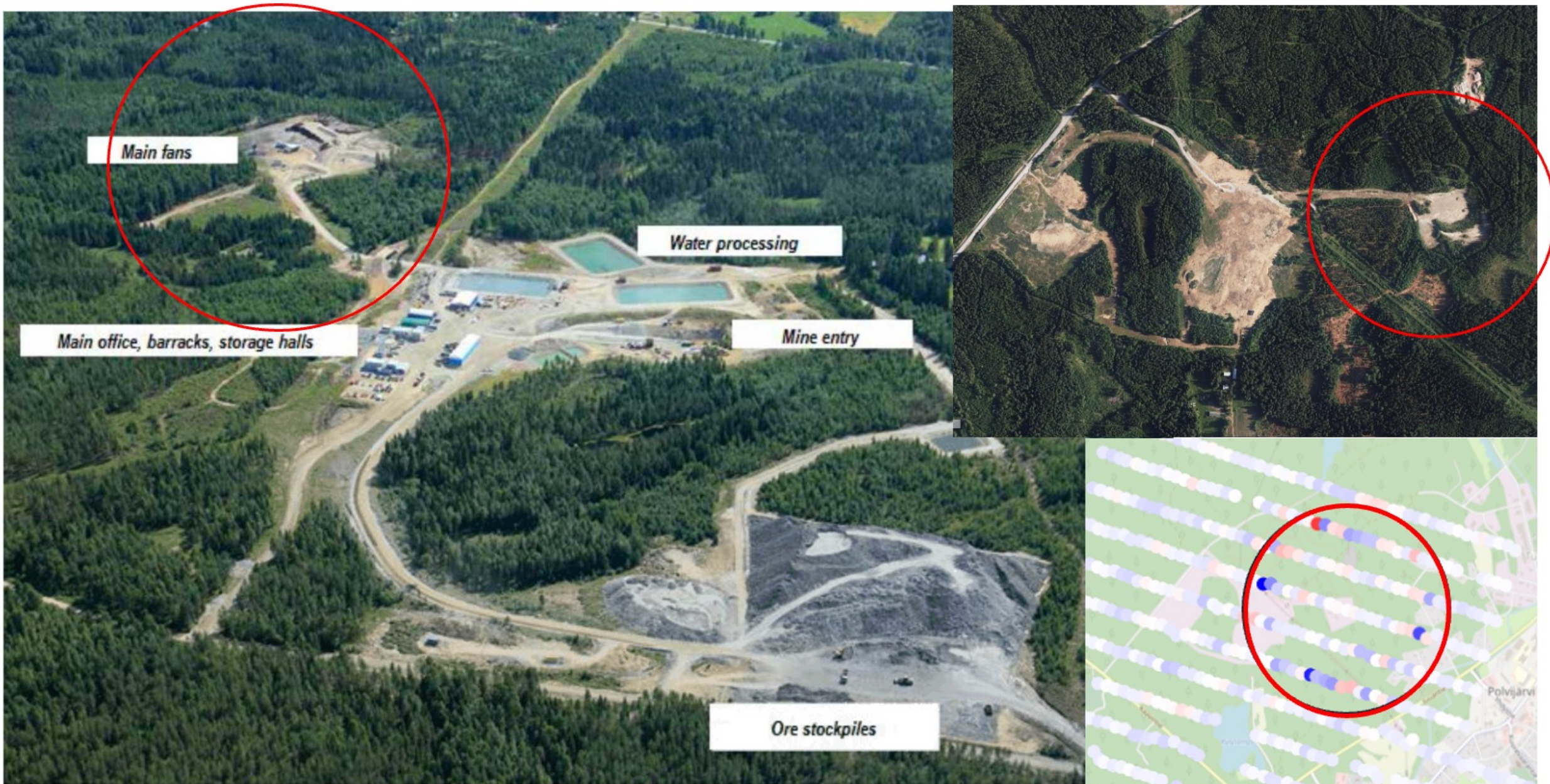
Figure 14. Surface infrastructure of Kylylahti mine.
