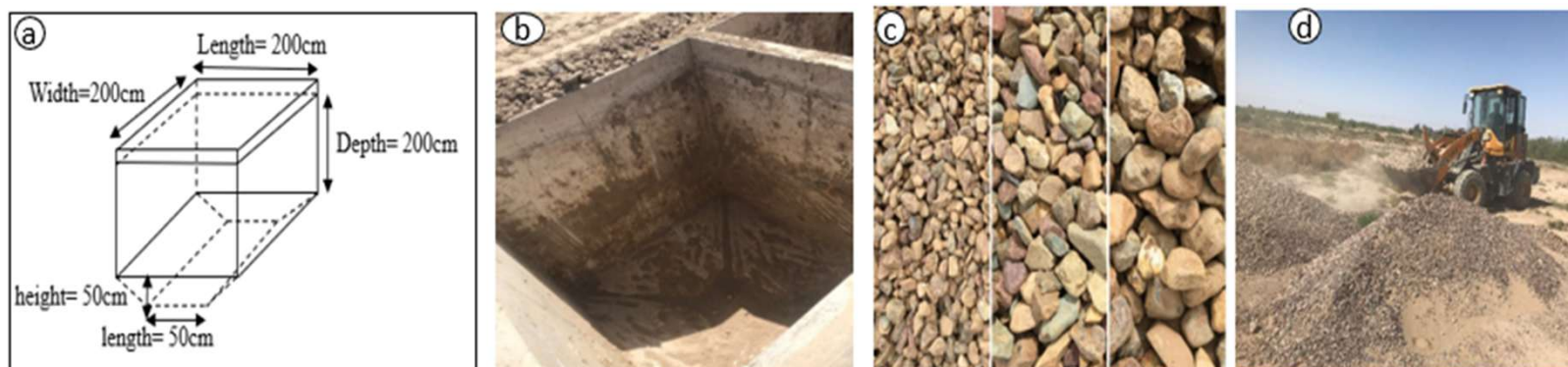
a) Sketch view of the plot b) Empty field plot , c) Gravels size d) Caterpillar machine with gravel
