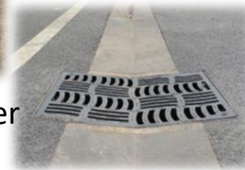
Storm drain / Gully
