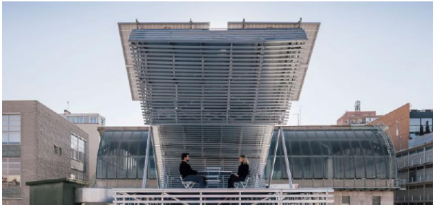
Photovoltaic shade, Madrid (ES)
