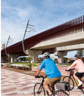
Level Crossing Removal Project – Carrum, Seaford and Kananook, Melbourne (AU)
