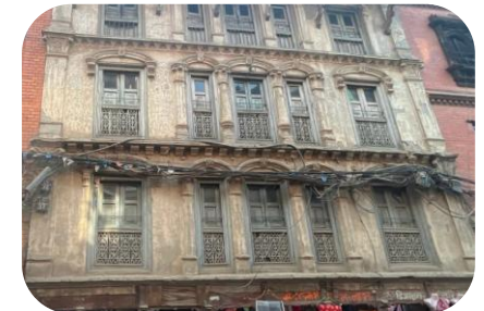
2. Old House Structure
