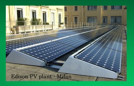
Production [kWh] = irradiance [kW/m<sup>2</sup>] \*h\* 17% \* 75% \* total area [m<sup>2</sup>]
