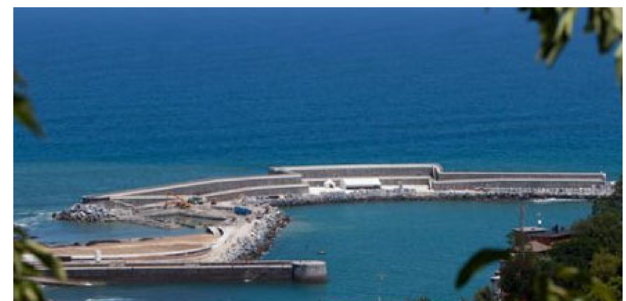
Figure 2: Aerial photograph of the Mutriku Wave Energy Plant
